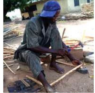
C. Construction of the Left Arm Stand
