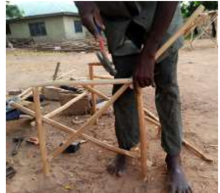
F. Construction of the Backrest with the Two Back-posts
