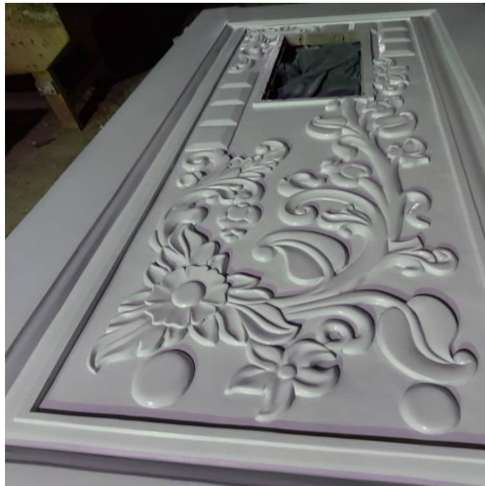
Figure 9: Application of primer on the door
